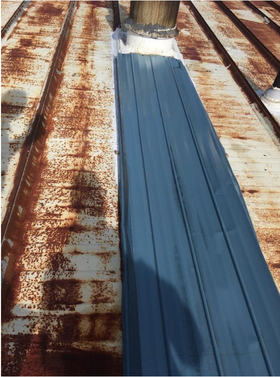
Chimney's to be removed shown above. Metal panel to be removed shown above.
