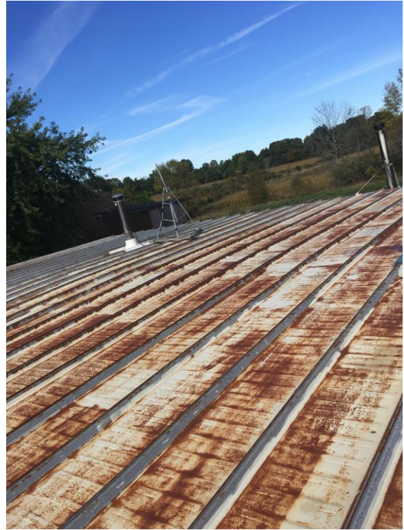
Chimney's to be removed shown above. Metal panel to be removed shown above.
